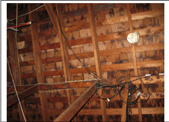
Picture 6 Cedar shingles roof decking
